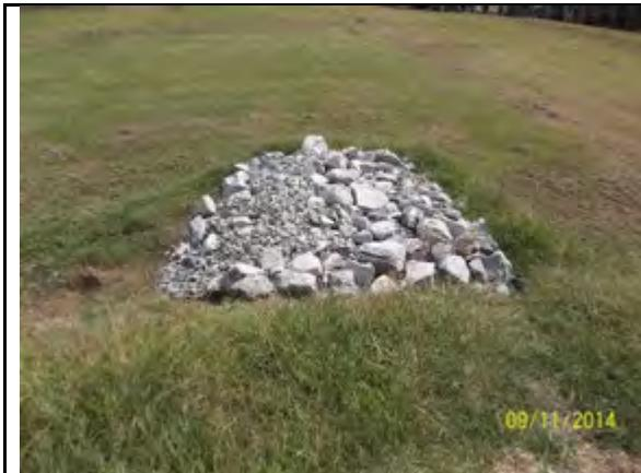
Fig. 1 – Check dam along east side of building that requires shaping revisions (view-east).
