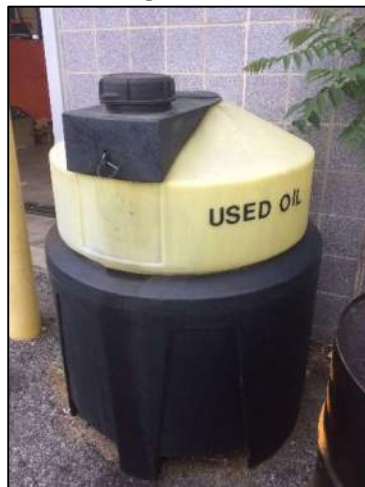
3: Used Oil Storage
