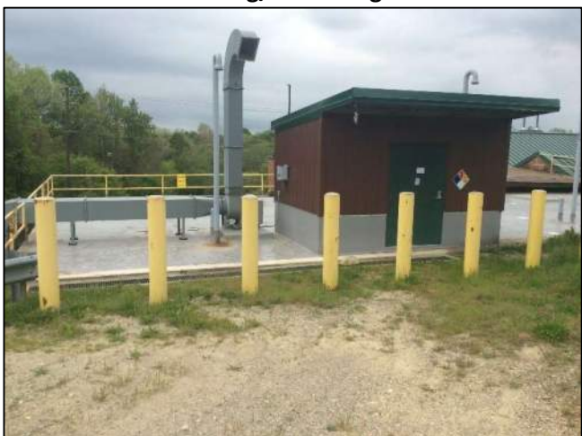
11: Heating Plant (boiler backup fuel storage)
