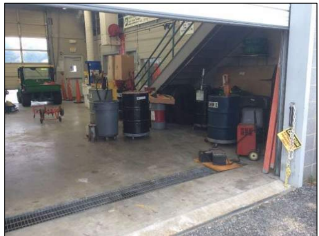
4: Maintenance Bay (with trench drain)
