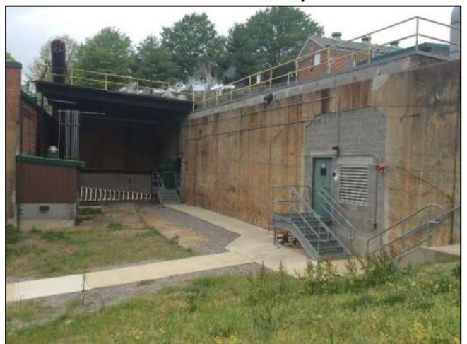
12: Heating Plant (boiler backup fuel storage)
