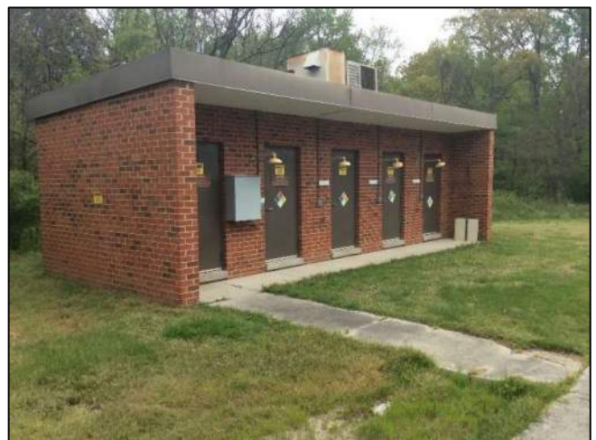
18: Hazardous Waste Storage Area
