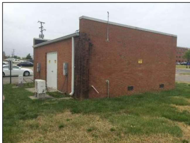
17: Hazardous Waste Storage Area
