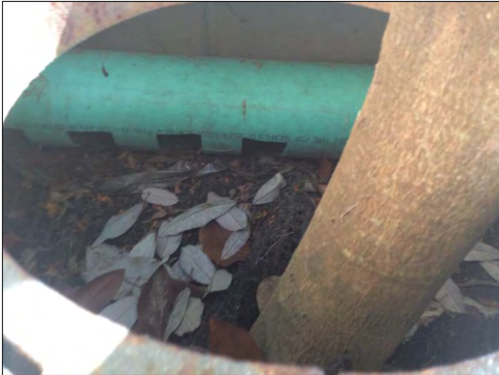
Stone Replacement within Roof Inlet Filterra (Typ.)
