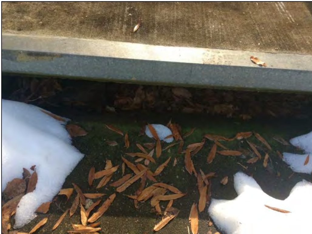
Stone Replacement within Curb Inlet Filterra (Typ.)
