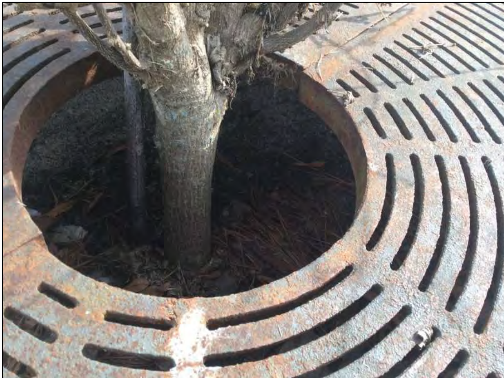
Netting in Need of Replacement (Typ.)
