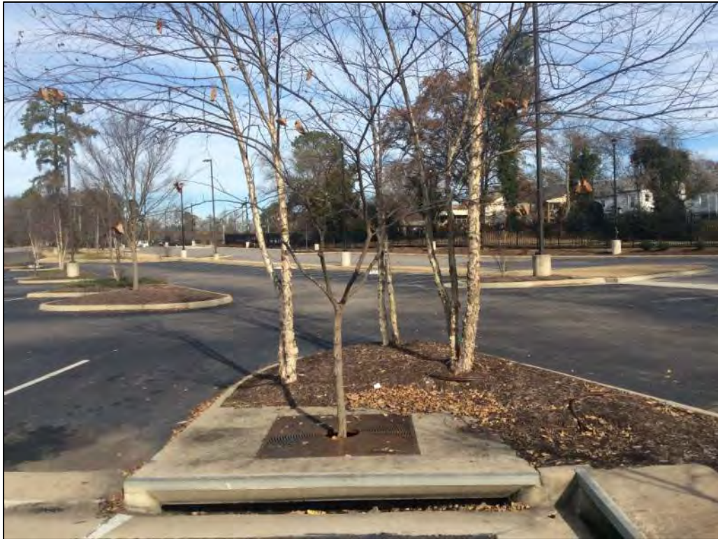
BMP 7-13, 41-44: Curb Inlet Filterra (Typ.)
