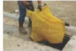
Slide SiltSack® over opposite side of grate.
