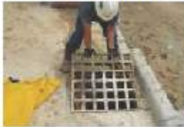
Remove grate from catch basin.
