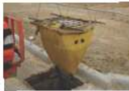
Removed SiltSack® is now ready for cleanout.
