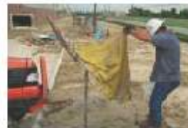
To clean SiltSack® attach rebar through empty loops at bottom and lift to empty.
