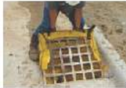
Slide SiltSack® over one side of grate.
