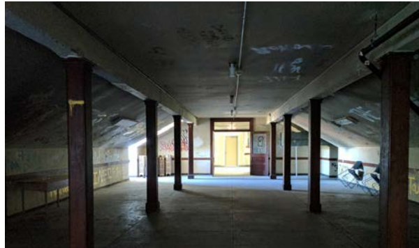
Existing Fourth Floor of Seward Hall
