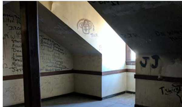
Existing Fourth Floor of Seward Hall
