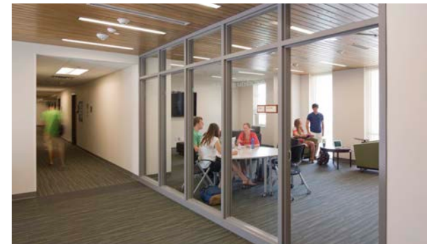
Example of Glass Partition between Corridor and Meeting Room
