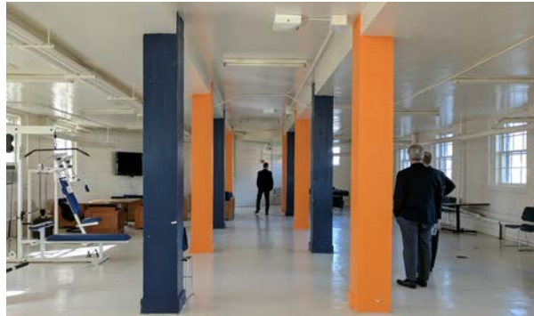
Existing Basement in Williams Hall
