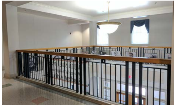
Existing Second Floor Balcony
