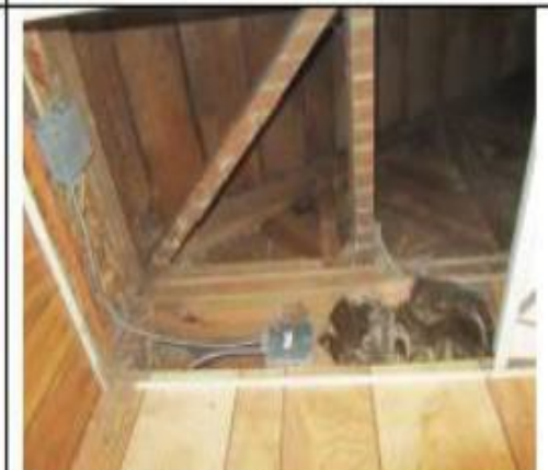
Original Interior gutted w/ energy inefficient Renovation
